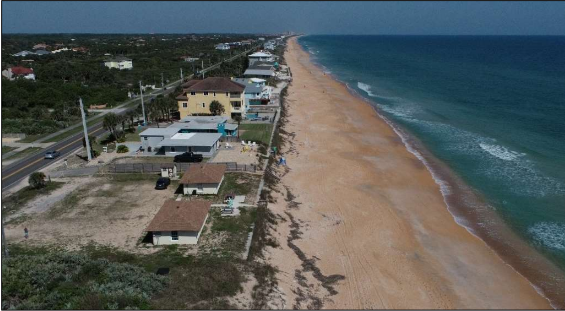
Figure 2.9: Looking north along the seawall in Painters Hill, 18 April 2019.
