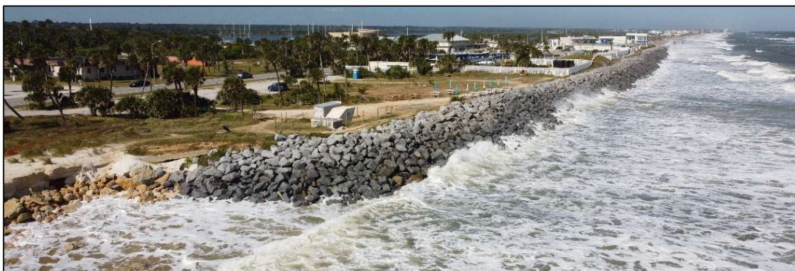
Figure 2.7: The revetment at Marineland, R-1 to R-2.3.
