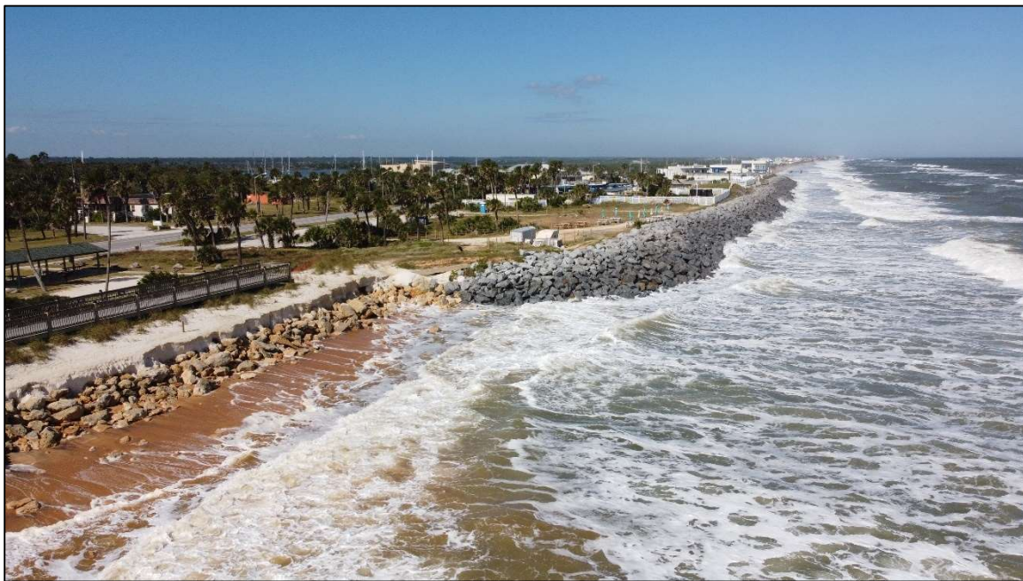
Figure 4.2: Typical conditions beach and dune conditions along Area 1 (09 November 2021); Marineland.
