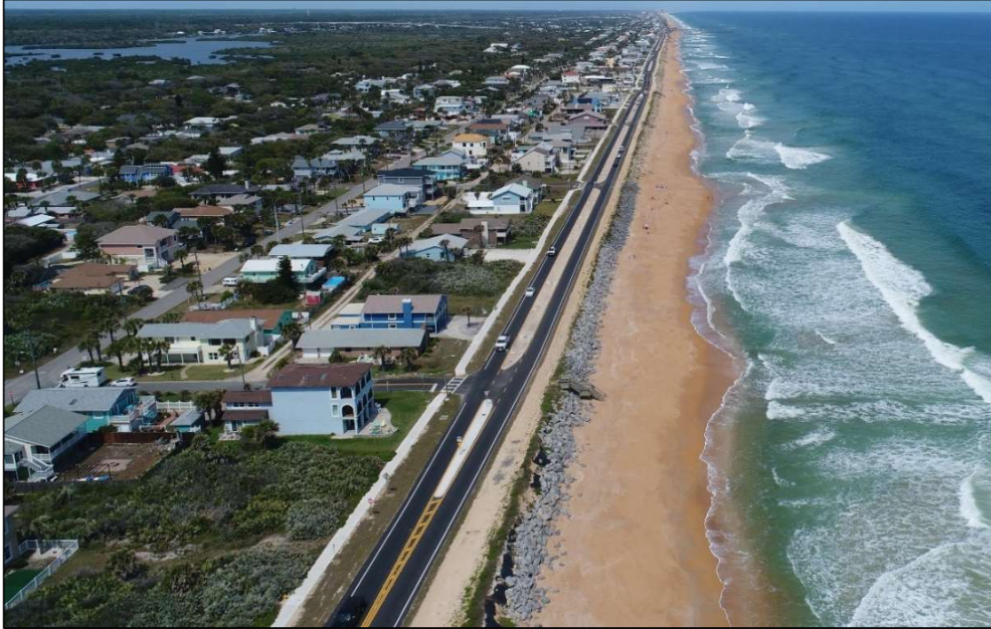
Figure 2.12: A portion of the revetment along SR A1A, looking north from R89.5, 18 March 2020.
