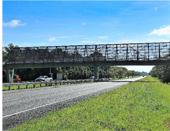
Flagler Greenway Pedestrian Bridge
