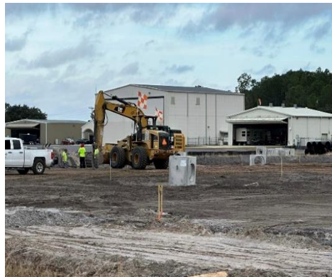
Flagler County Executive Airport – growth through construction of new T-Hangars
