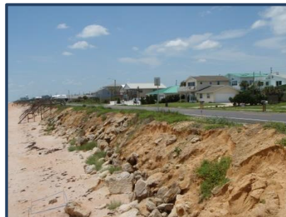
Before Mitigation and After Mitigation
