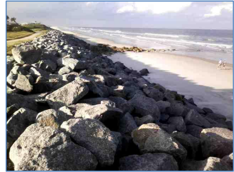
Coastal structures can reduce flooding and stabilize the shoreline
